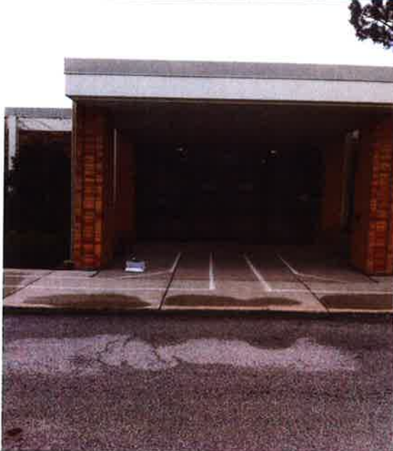
View outside Subject Building, location for Sample 21863589.
